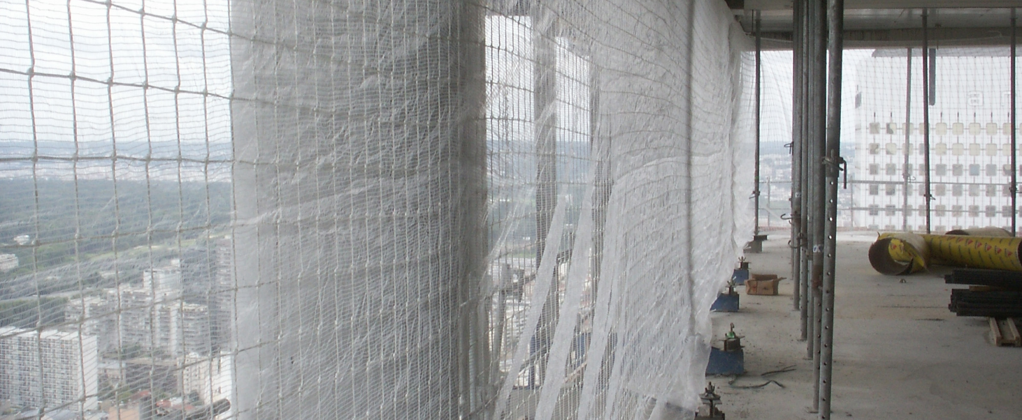
Normachute - vertical installation
